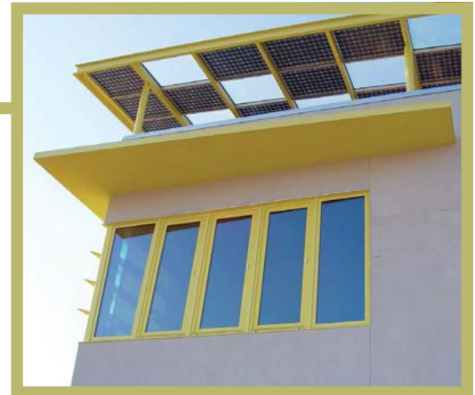
Overhangs provide some protection from the summer sun, although heat-blocking shades are also used.
