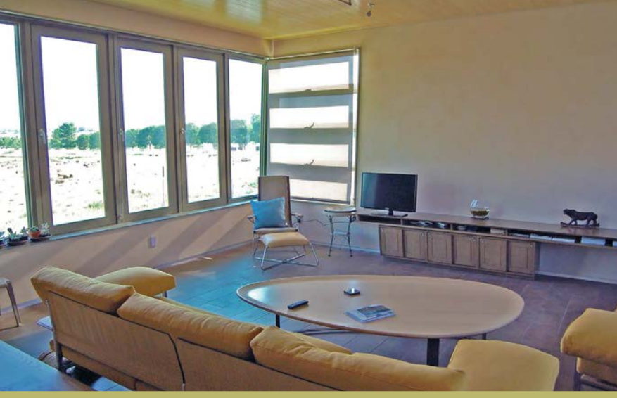
Ample south-facing glazing admits direct solar gain, which is absorbed by the concrete floor. This heat energy, stored in the floor, is released when interior temperatures drop below the floor's temperature.
