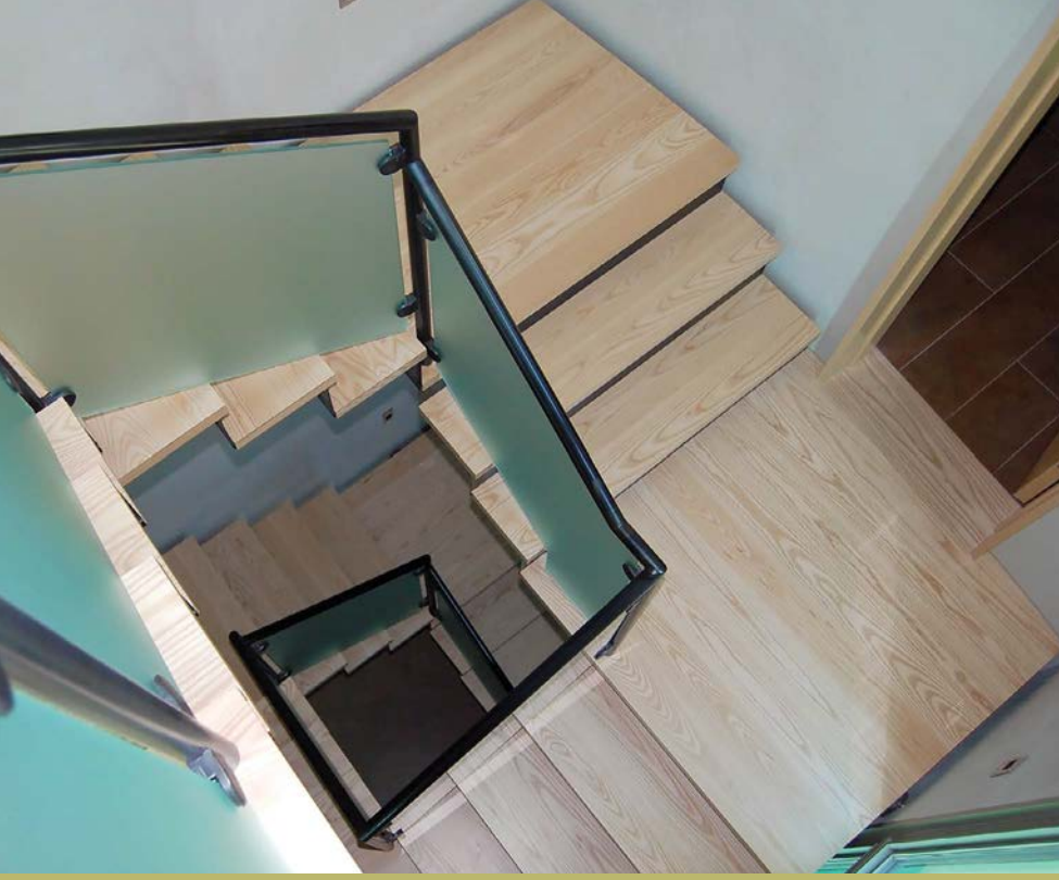
With slotted steel risers, the home's central staircase acts as a giant vertical return, feeding the return air grille on the ground level.
