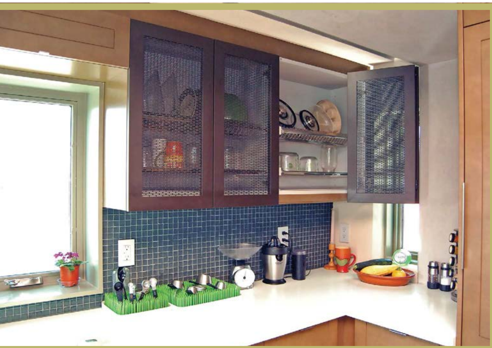
A clever open-air drying rack, incorporated into this cabinet, eliminates the energy used to heat-dry dishes in a dishwasher. The countertops are made of Durat, a material that contains post-consumer industrial plastic.
