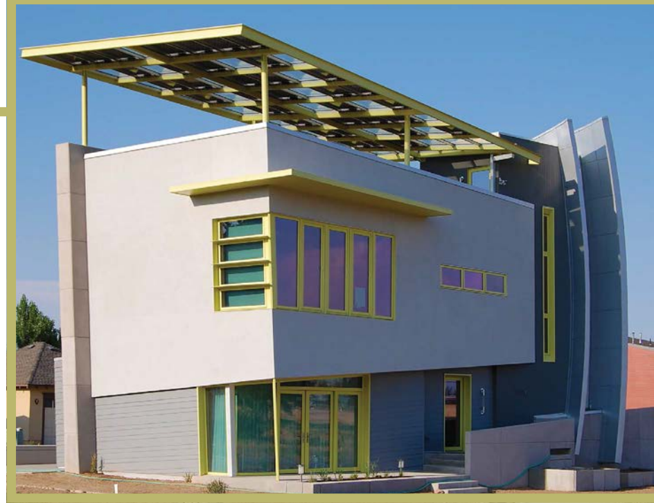
The home's south face was designed to capture direct solar gain in the winter, reducing the need for supplemental space heating. A 7.02 kW awning-mounted PV system is anticipated to offset all of the home's electricity use.
